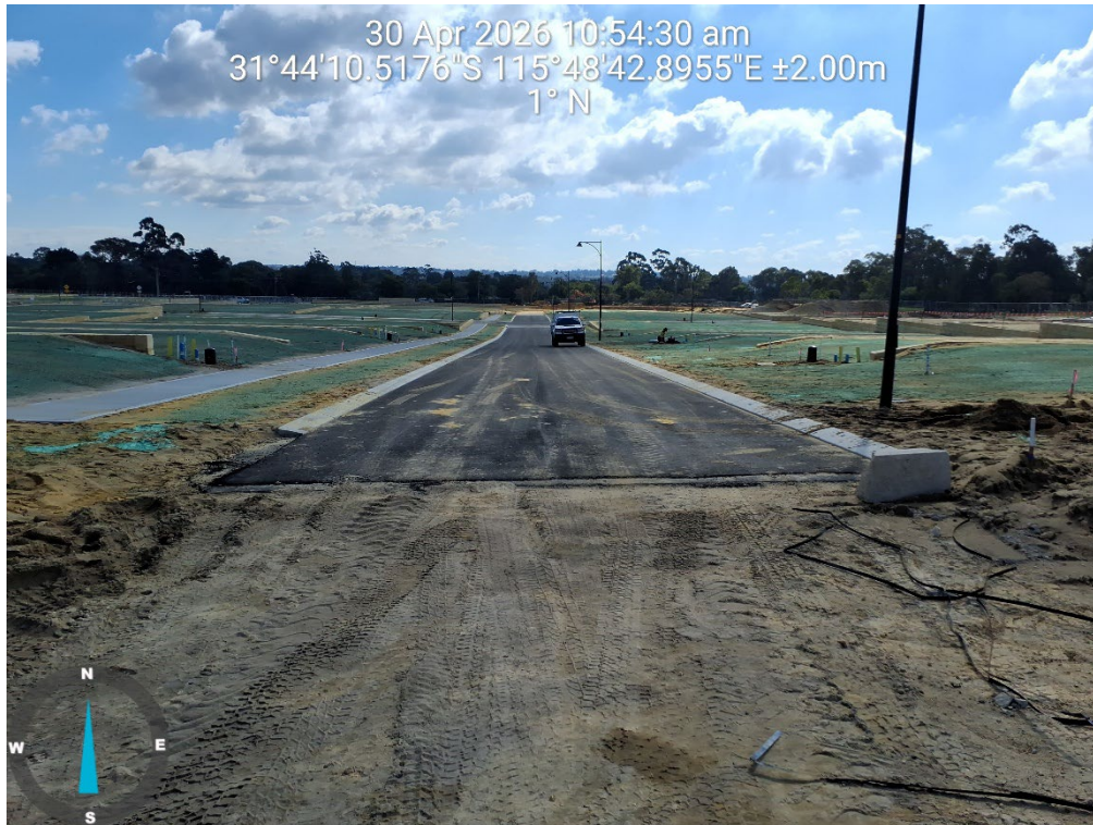
Plate 3: Roads within the subject site which have been constructed during Stage 1 development.
