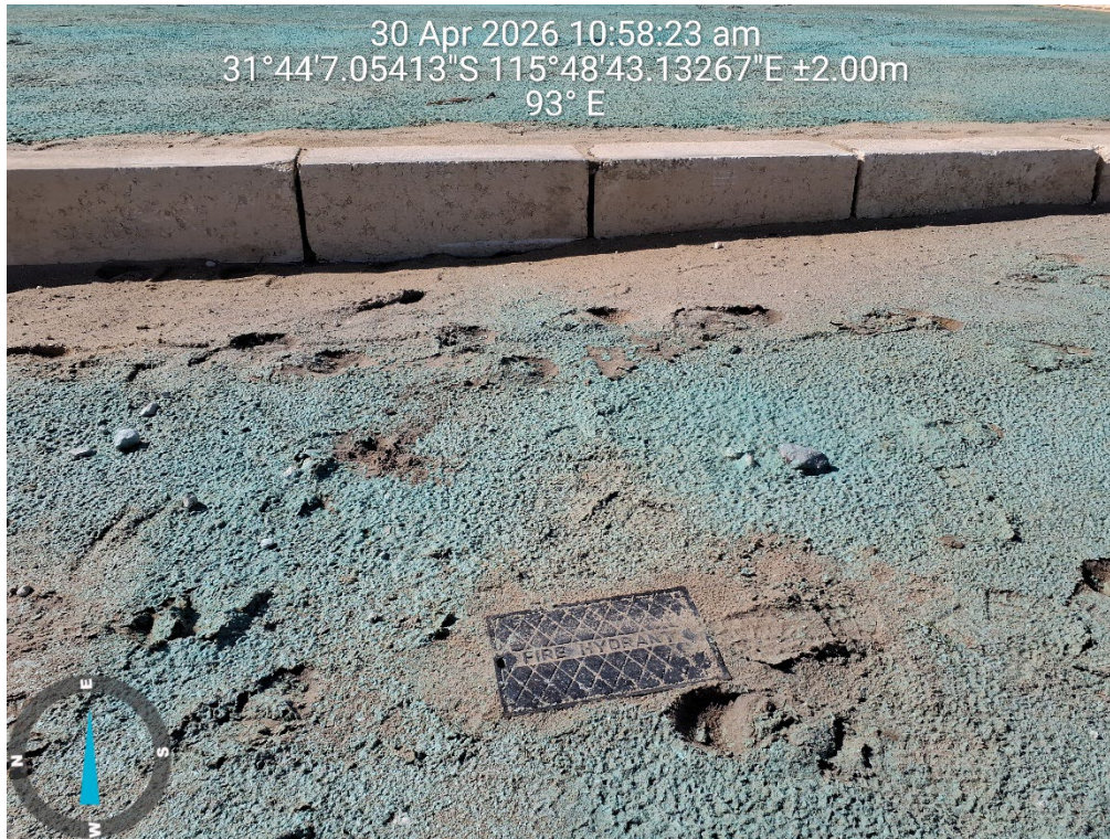
Plate 7: Hydrants installed within Stage 1 of Valencia Estate.
