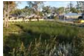
Vegetated stormwater detention basin with reed and sedge planting
