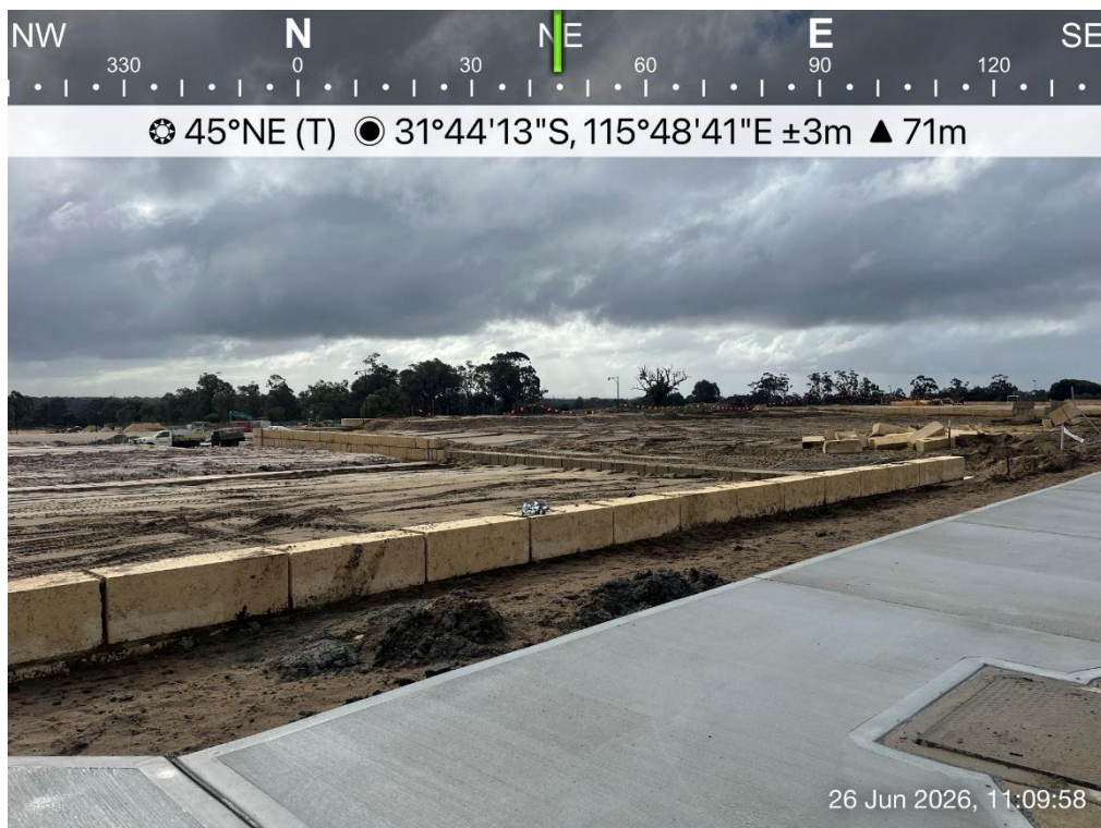
Plate 2: Areas surrounding the subject site which are devoid of vegetation.
