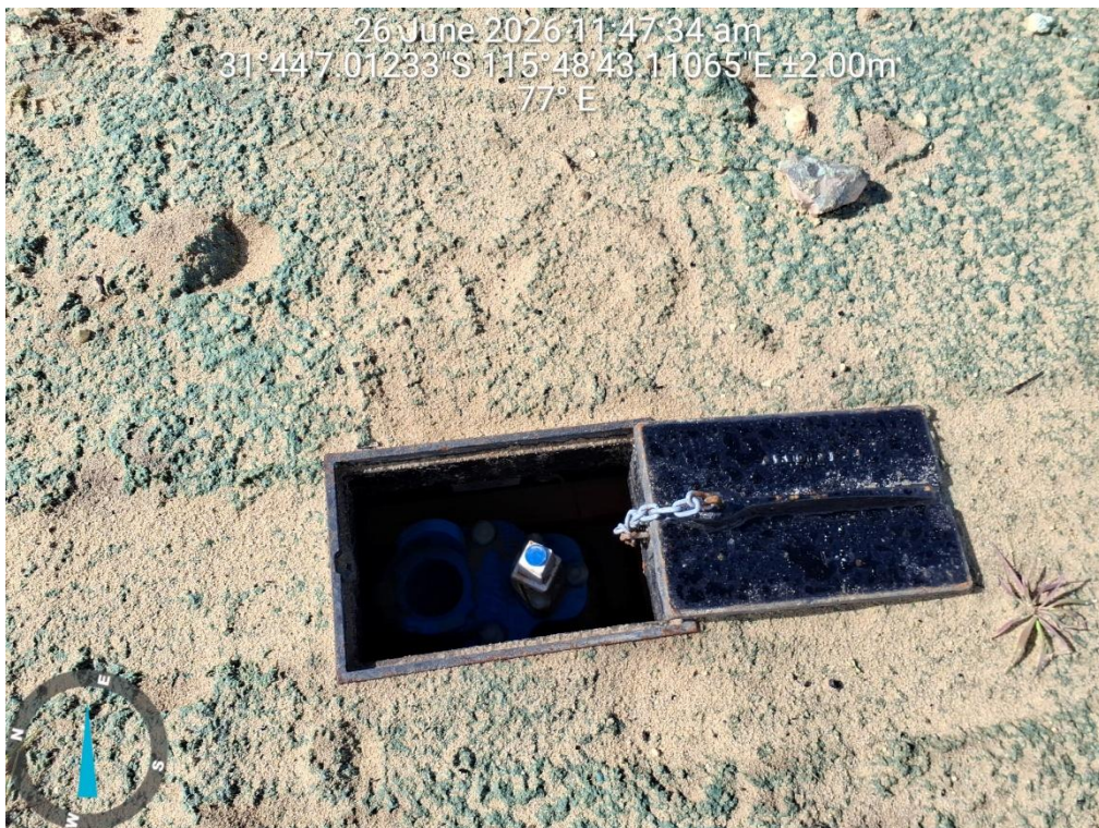
Plate 5: Hydrants installed within Stage 1B of Valencia Estate.
