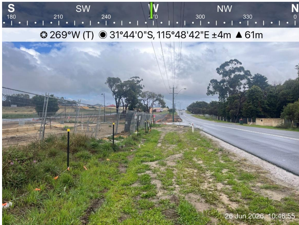
Plate 1: Vegetation maintained to Asset Protection Zone standards within the Caporn Street road reserve.
